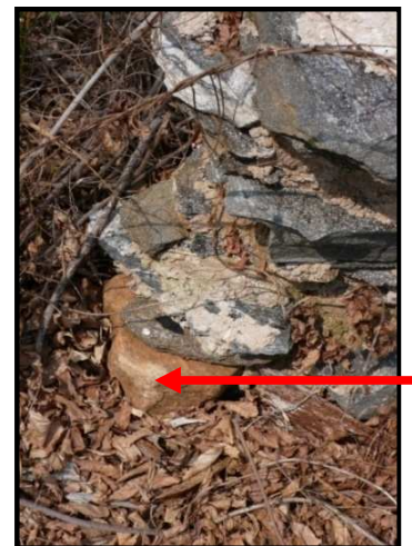
Figure 7: Field stone at base of pier
