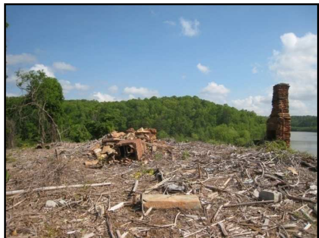
Figure 2: Close-up view of the house site facing north– note standing chimney on the right (east) and collapsed chimney on the left (west)
